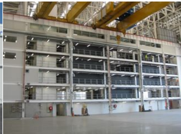
Internal Pre-Out fit building
