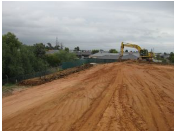
Cranbourne (VIC) - Clay capping – pre liner
